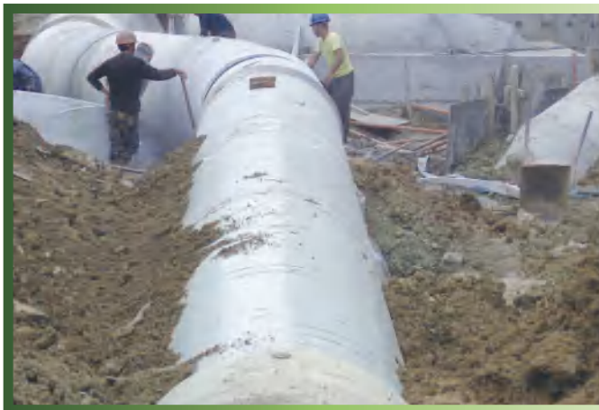
DN1200mm PN0.6MPa FRP Pipeline Project supplying water from Laiwu Xueye Reservoir To Laigang Specification :DN1200mm, PN0.6MPa
