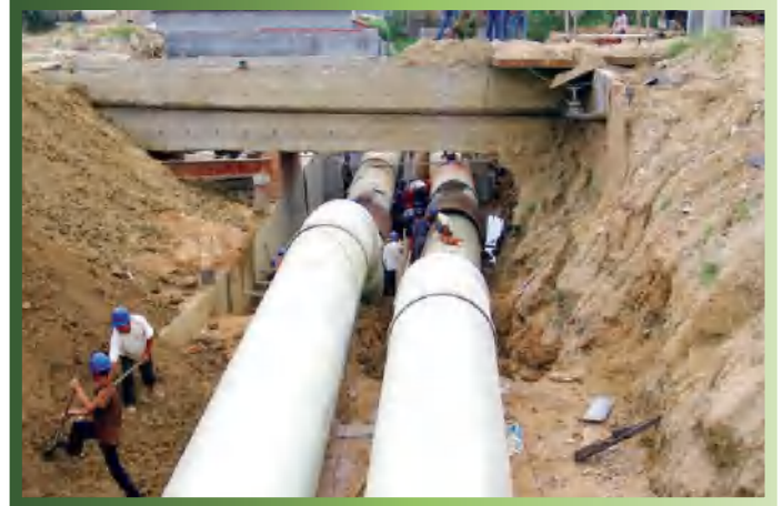
GRP Pipe Network Project for Seawater Desulfuration in Shougang-owned Electric Power Plant Specification: DN300mm-DN1200mm, SN10000N/m 2
