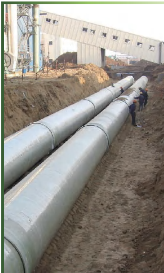
DN1600mm SN10000N/m 2 Circulating Water and Cooling Water FRP Pipeline Project for Sinopec Shengli Electric Power Plant Specification: DN1600mm, SN10000N/m 2
