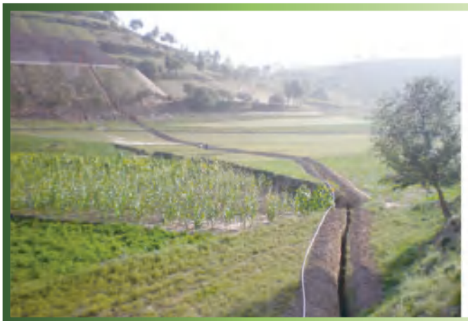
DN40mm PN25MPa High-pressure GRE Pipeline Water Injection Project for Yanchang Oilfield Dingbian Production Plant No.3185 Wuxingzhuang Station Specification: DN40mm, PN25MPa
