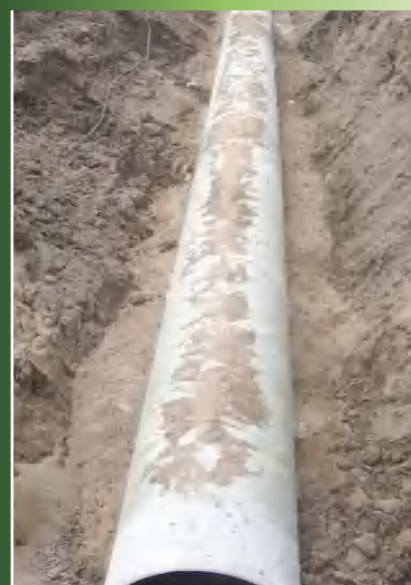
河南新乡自来水供水玻璃钢管网工程 规格型号: DN800mm、PN0.8MPa Henan Xinxiang Drink Water Supply GRP Pipe Network Project Specification: DN800mm,PN0.8MPa
