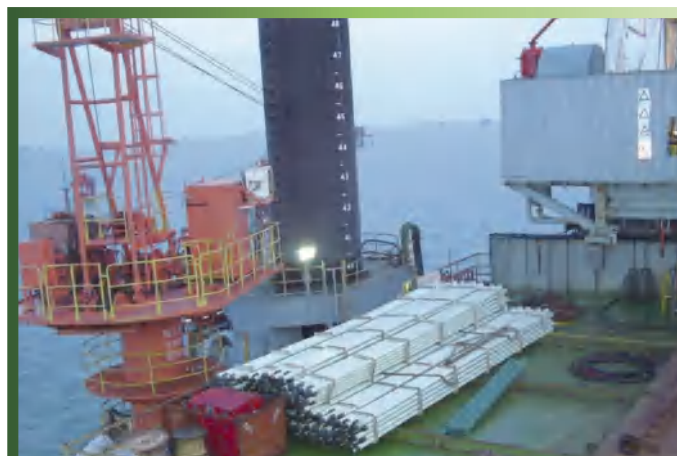
High pressure GRE downhole tubing transported to the 8th Offshore Platform
