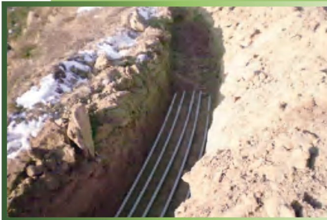
DN40mm-DN150mm PN5.5MPa-PN25MPa GRE Pipeline Water Injection Network Project for Yanchang Oilfield West Block Yiwu No.1 Water Injection Station Specification: DN40mm-DN150mm, PN5.5MPa-PN25MPa
