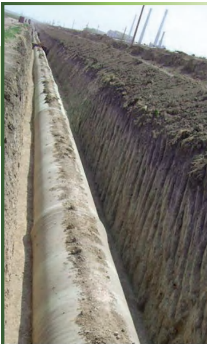
DN1400mm-DN1600mm SN10000N/m 2 FRP Pipeline Project for Interception of Sewage from Wastewater Treatment Plant at Zibo Zhoucun District North Suburb Specification: DN1400mm-DN1600mm, SN10000N/m 2
