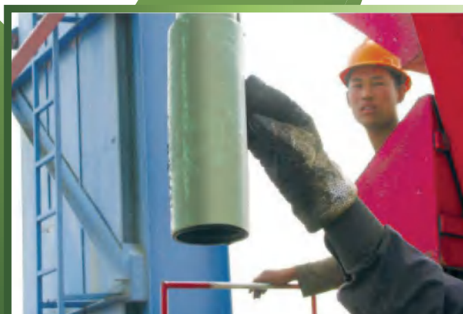
High pressure GRE downhole tubing being run in hole at Yong 35-10 well
