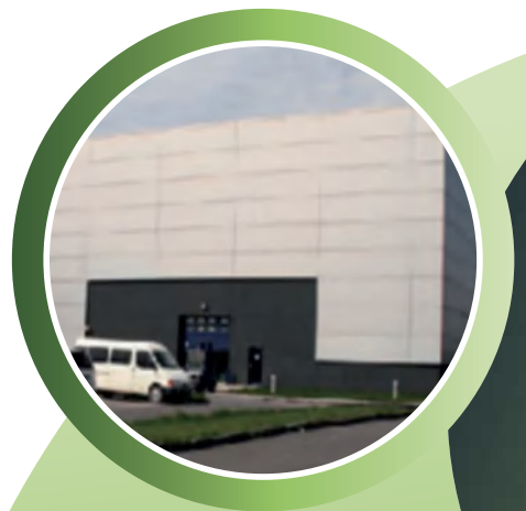
Building curtain wall
