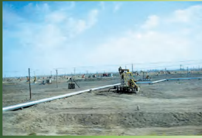
GRP Water Supply Project for Tahe Oilfield in Xinjiang Specification: DN300mm-DN500mm, PN1.6MPa Length :110km
