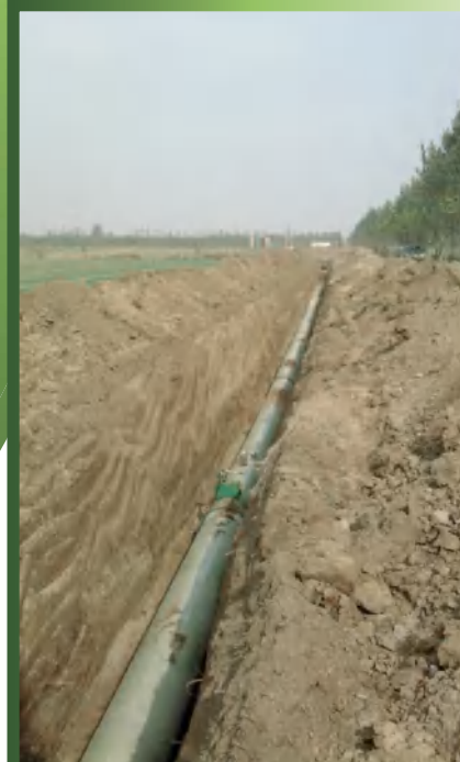
GRP Pipe Network Project for Seawater Desulfuration in Shougang-owned Electric Power Plant Specification: DN300mm-DN1200mm, SN10000N/m 2
